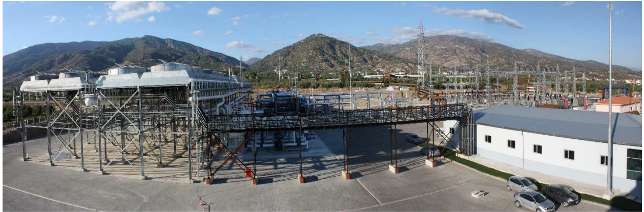
Figure 22 : Sight of the geothermal power plant of Pamukören in Turkey equipped with two ORC turbines of 25 MWe atlas Copco Energas (© Verkis). To the left, we distinguish the drum kits of ventilators for the cooling by air.
