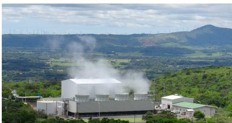
Figure 5: Cooling system with cooling towers of the power station in Miravelles, in Costa Rica (©Biotope, 2014).
