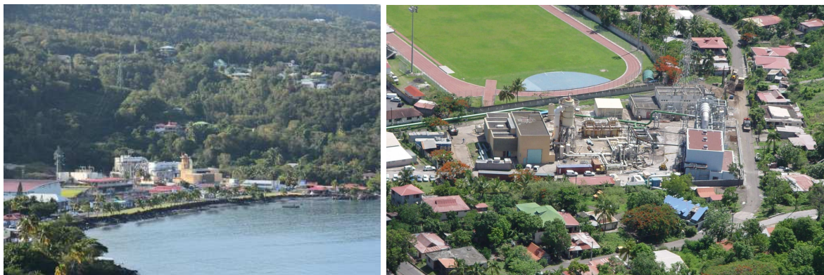
Figure 3 : View of the geothermal plant of Bouillante, Guadeloupe, implanted in the city of Bouillante (©CFG Services).
