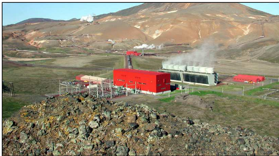
Figure 20 : The geothermal power plant of Krafla in Iceland ( 60 MWe) equipped with a steam turbine with double flash (© Verkis).
