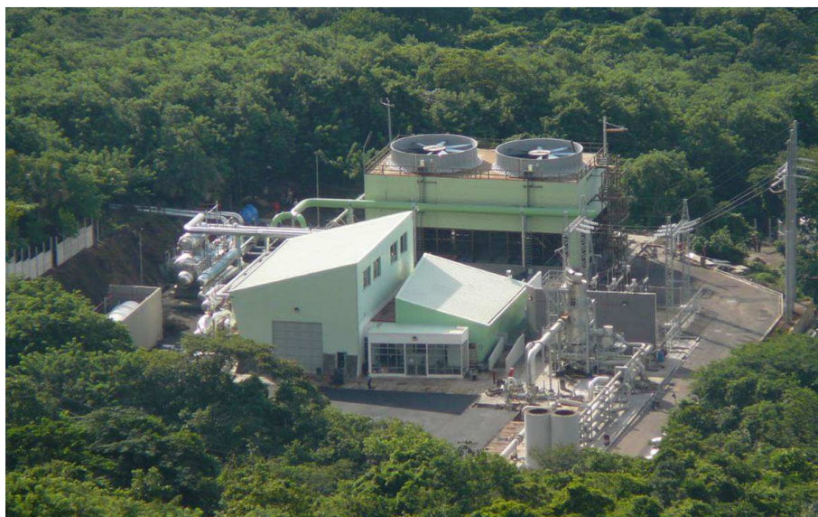
Figure 3: Berlin's geothermal power plant in Salvador, with a capacity of 109 MWe (sources: Verkis).
