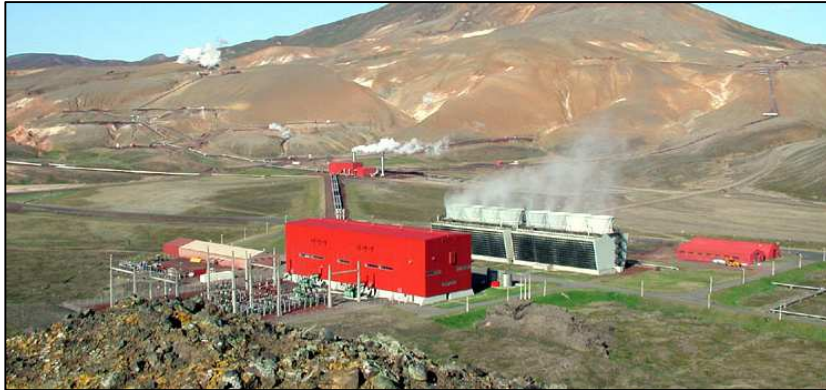
Figure 2: Inverse flow cooling tower at the geothermic power stations in Krafla in Island. (60 MWe) (©Verkis).
