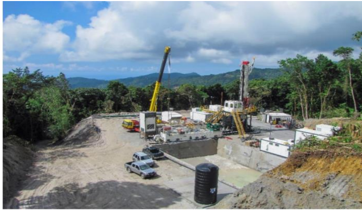
Drilling Site – Dominica
