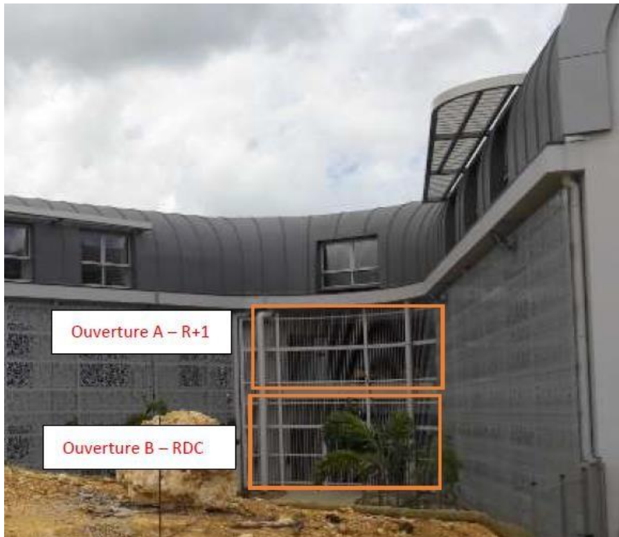
External view of inter-building passageways (open on the ground and first floors – closed on the second floor)
