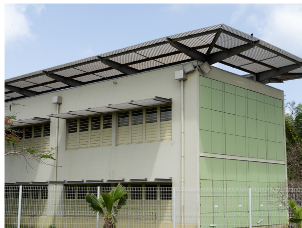
FIGURE 5. Examples of eaves and caps.
