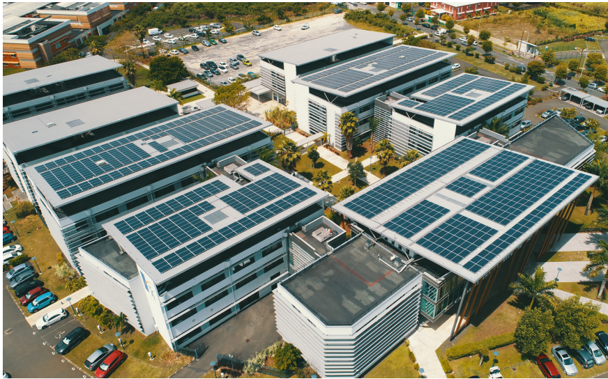
FIGURE 26. Rooftop PV system.
