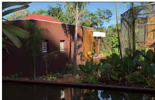
Shading effect induced by the vegetation on the north façade
