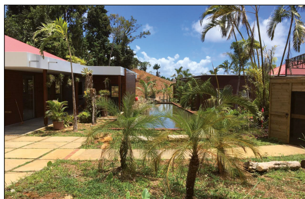
View of roof eaves that form caps
