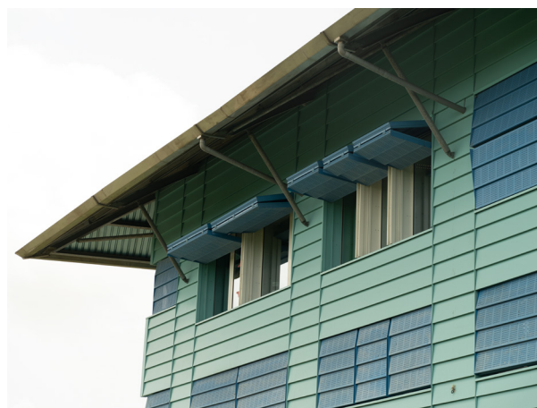
FIGURE 2. Example of solar shading of glazed walls.
