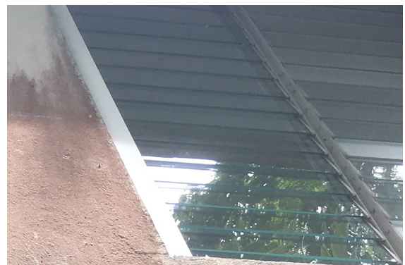
FIGURE 20. Example of a non-airtight blind. In the closed position, a space can still be seen between the slats and airtightness is not provided.
